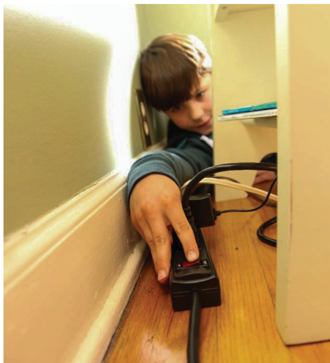
Surge protectors are sold at local stores. Contact a certified electrician about whole-house surge protectors. PHOTO COURTESY OF TOUCHSTONE ENERGY COOPERATIVES
